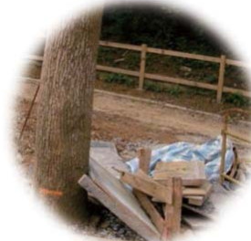
Don't undertake works within the tree protection zone 切勿在樹木保護範圍內進行工程
