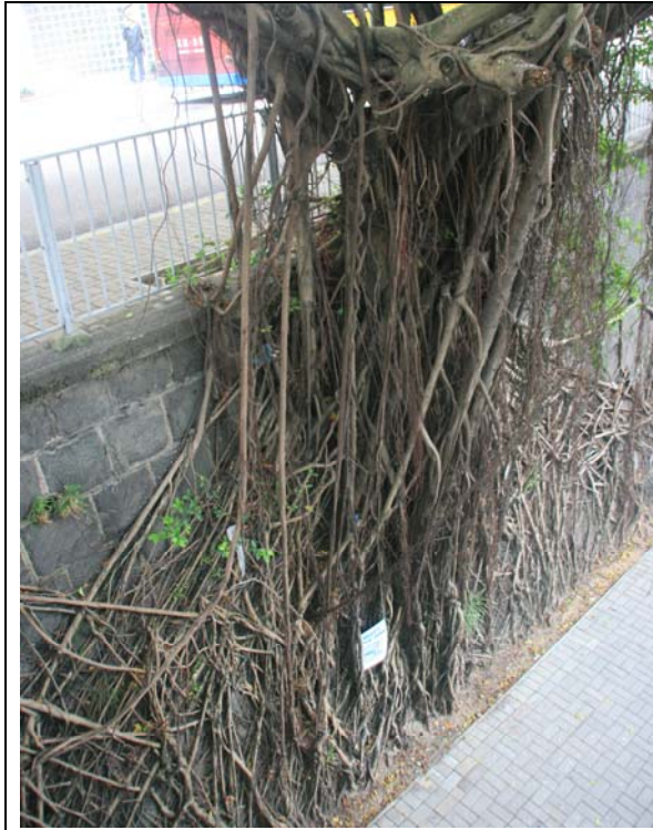
Photo No. 6 – Provision of rooting areas at the toe of the retaining wall
