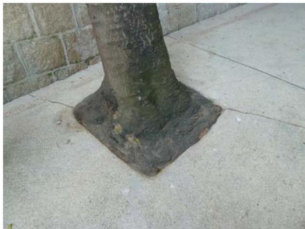
Fig. 6 A bad example showing a tree surrounded by concrete around the root collar
