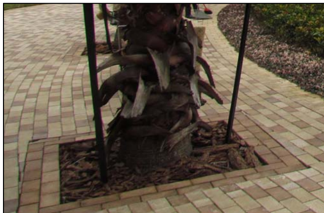
Fig. 9 Permeable paver blocks on sand base
