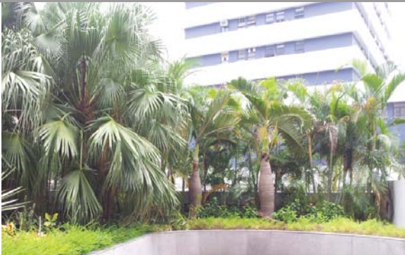
位於土木工程拓展署大樓的平台花園 Podium planting at Civil Engineering and Development Building
