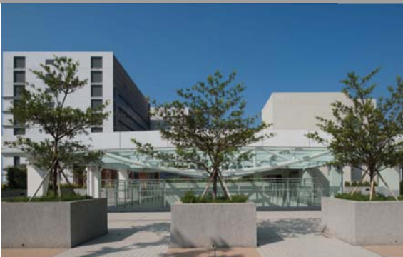
位於深水埗歌和老街特殊學校的屋頂綠化 Green roof of Special School at Cornwall Street, Sham Shui Po
