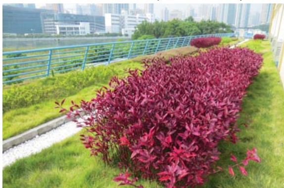
粗放型屋頂綠化 Extensive green roof
