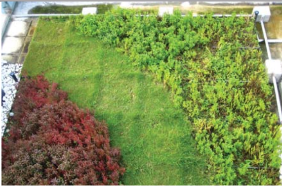
位於水務署設施上的屋頂綠化 Green roof at Water Services Department's facility
