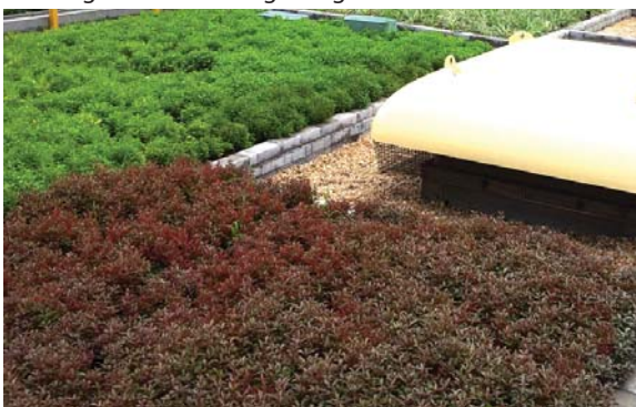
位於渠務署設施上的粗放型屋頂綠化 Extensive green roof at Drainage Services Department's facility
