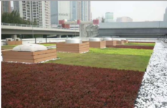
位於水務署設施上的屋頂綠化 Green roof at Water Services Department's facility
