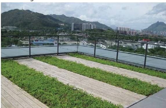
位於屏山天水圍公共圖書館的屋頂綠化 Green roof at Ping Shan Tin Shui Wai Public Library
