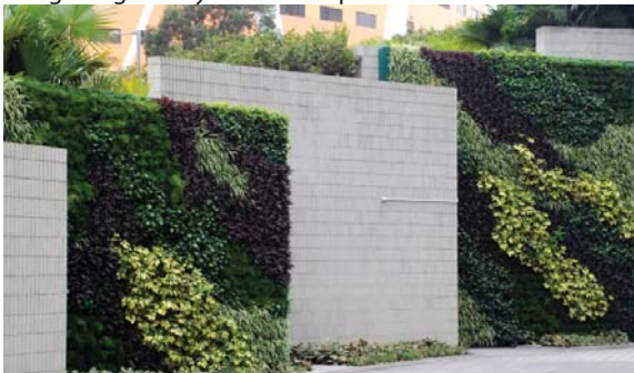
位於機電工程署總部外牆上配以多種植物作垂直綠化 Vertical greening with other plants at Electrical and Mechanical Services Department Headquarters
