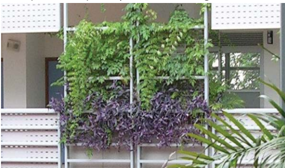
近鏡展示的層架式花槽 Close up of the stack planters at primary school in Tseung Kwan O
