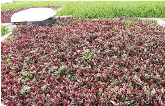
位於渠務署設施的粗放型屋頂綠化 Extensive green roof at Drainage Services Department's facility
