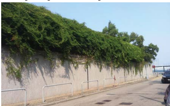
位於渠務署灣仔東基本污水處理廠的懸垂種植 Draping from wall top at Wan Chai East Preliminary Treatment Works of Drainage Services Department
