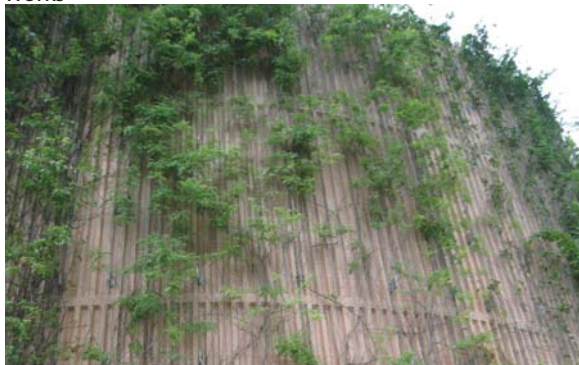
位於沙田污水處理廠的垂直綠化 Vertical greening at Sha Tin Sewage Treatment Works
