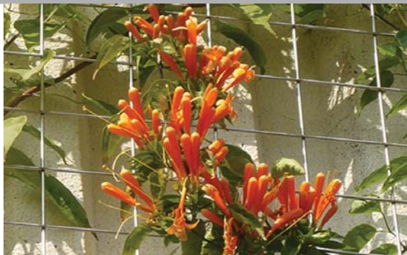
位於沙田污水處理廠的垂直綠化 Vertical greening at Sha Tin Sewage Treatment Works
