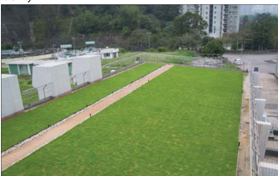
位於渠務署設施上的粗放型屋頂綠化 Extensive green roof of Drainage Services Department's facility
