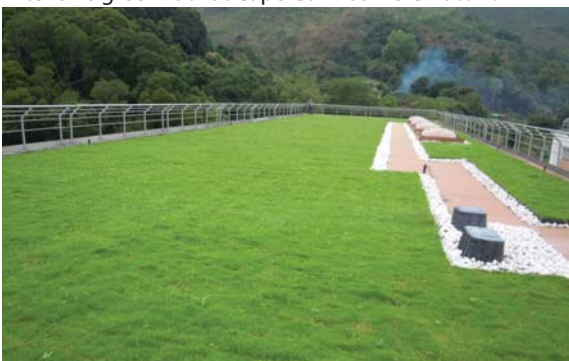
位於渠務署設施上的粗放型屋頂綠化 Extensive green roof of Drainage Services Department's facility
