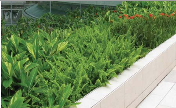
位於東涌游泳池場館的密集型屋頂綠化 Intensive green roof at Tung Chung Swimming Pool Complex
