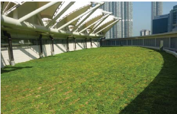
位於東涌游泳池場館的粗放型屋頂綠化 Extensive green roof at Tung Chung Swimming Pool Complex
