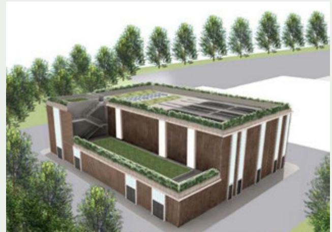
Ha Tsuen Sewage Pumping Station
