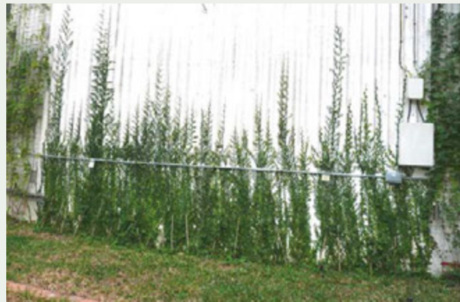
Tank 4 (testing of site factors and monitoring of cooling effect)
