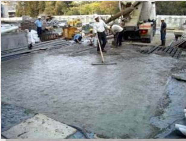
2. Pouring of concrete
