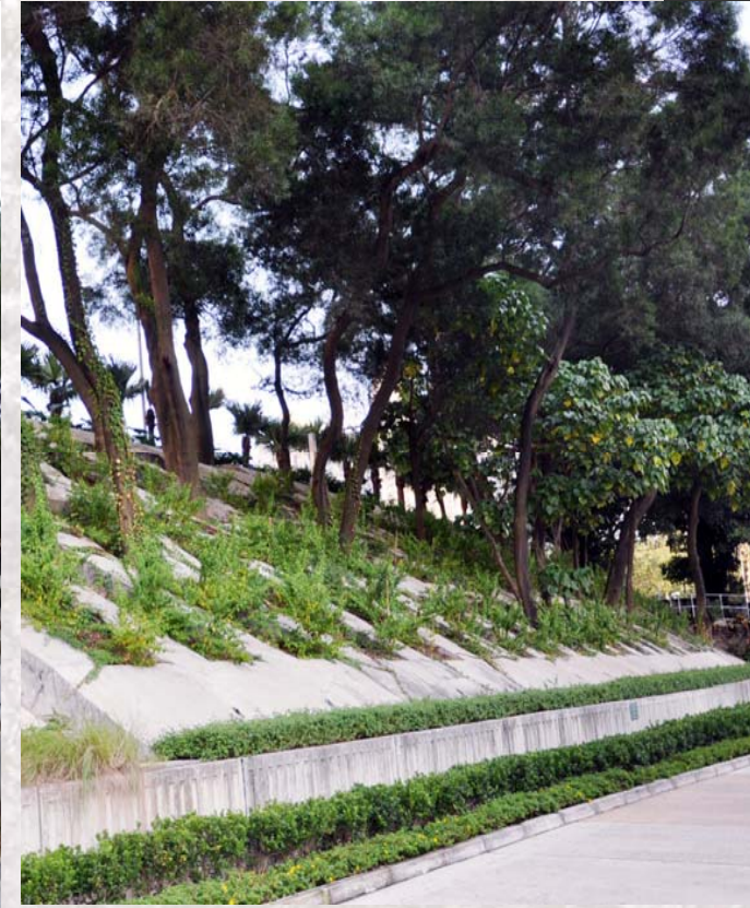
Concrete grillage completion
