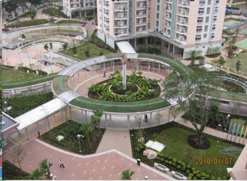
238M Roof greening on covered walkway with semi-automatic irrigation
