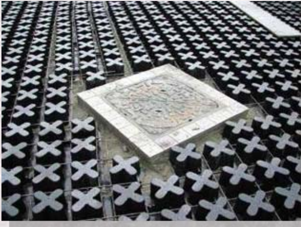
1. Laying of plastic former
