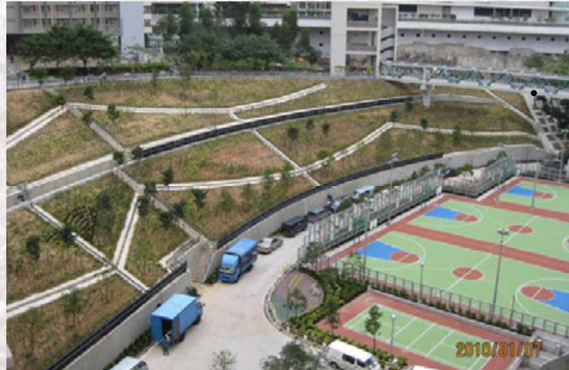
Reformed 30° fill slope
