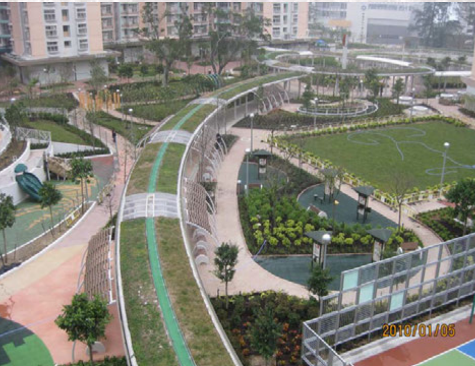
238M Roof greening on covered walkway with semi-automatic irrigation
