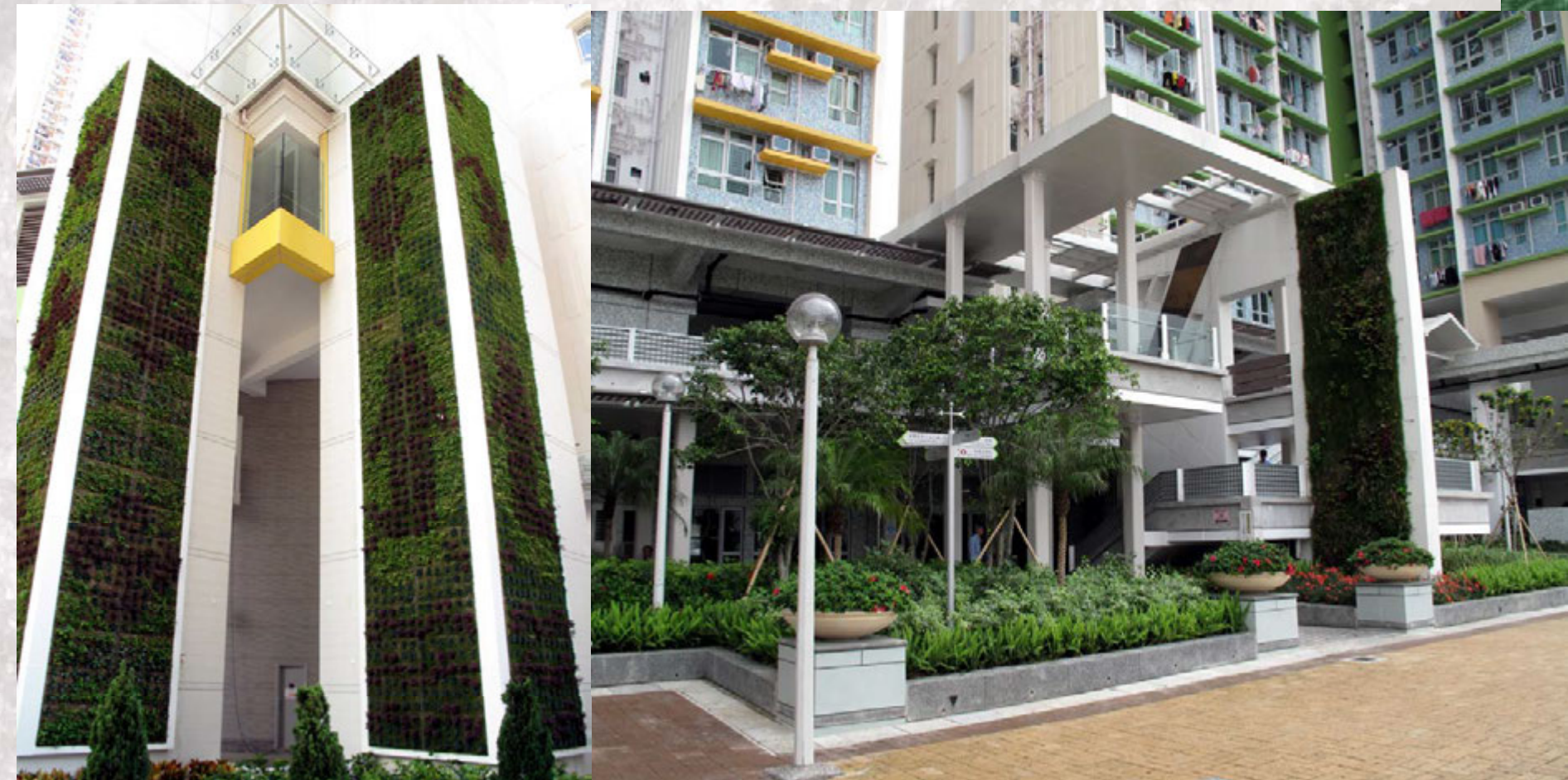
Yau Lai Estate (EHC Site) Ph.4
