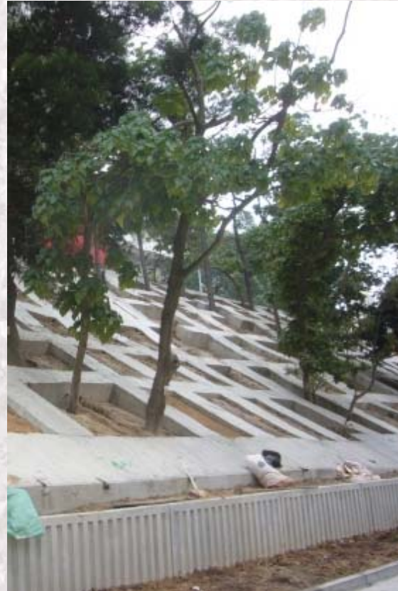
Concrete grillage with existing trees
