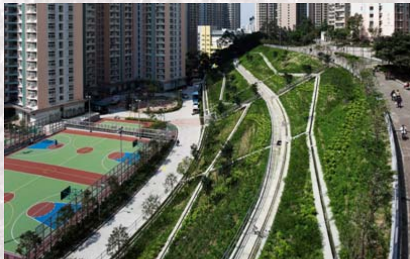
Full turfing on new slope
