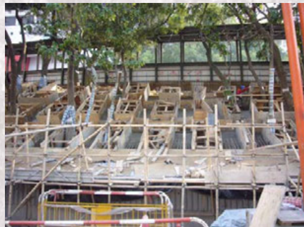
Concrete grillage during construction
