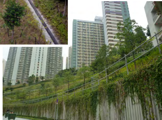
A vegetated cut slope with retaining wall at the toe (vegetation in a crest planter trailing down the wall)
