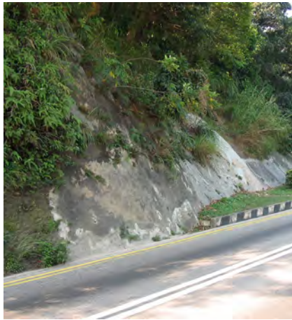
Before slope upgrading works
