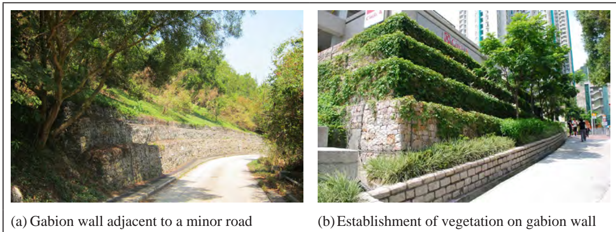
Figure 2.12 Use of Gabion Walls
