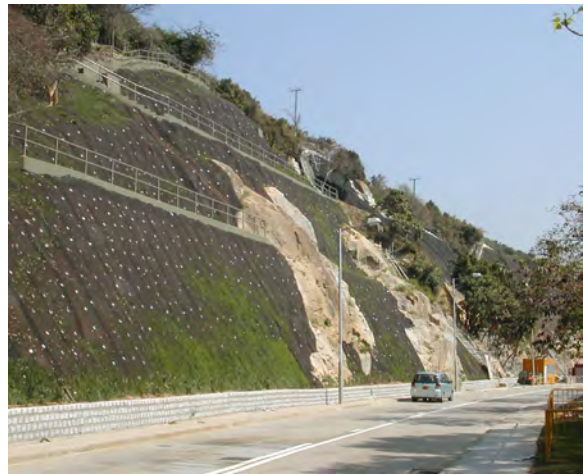
(b) Non-biodegradable erosion control mat
