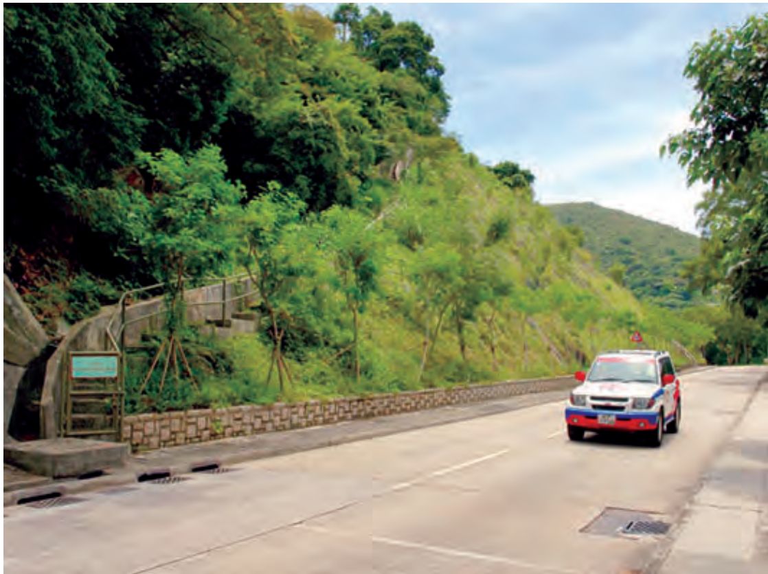
Cut slope planted with trees in a toe planter and access path contoured to reduce visual impact
