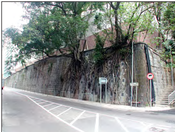
Completion of construction (2001)
