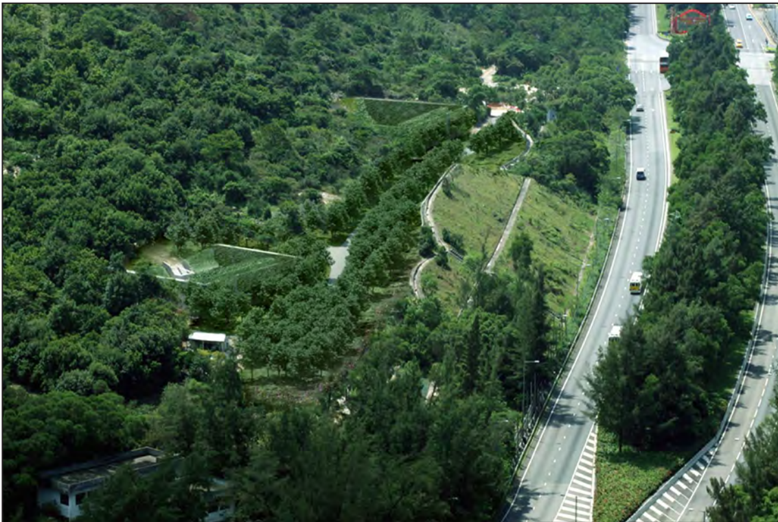
Photomontage showing an aerial view of the completed works
