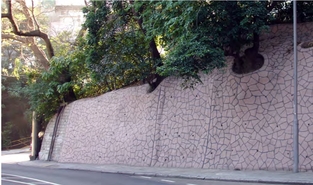
Use of a spray applied coloured masonry like finish to a hard surface
