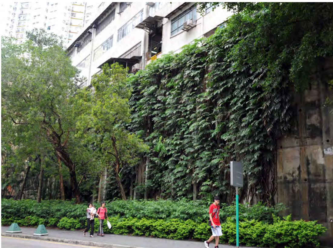
Climbers and screen planting at the toe to soften the appearance of a concrete retaining wall
