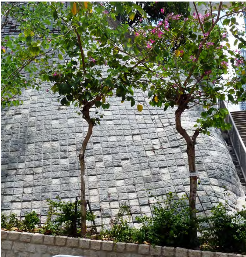
Use of patterned masonry blocks
