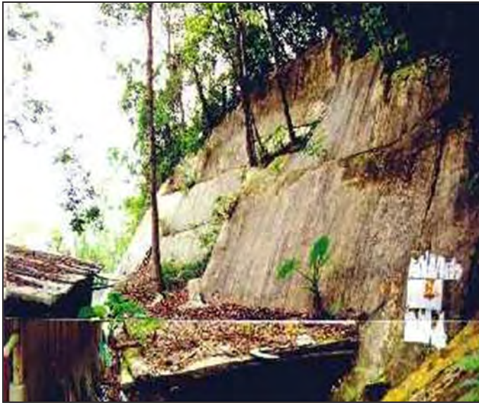
Slope before upgrading works (2000)
