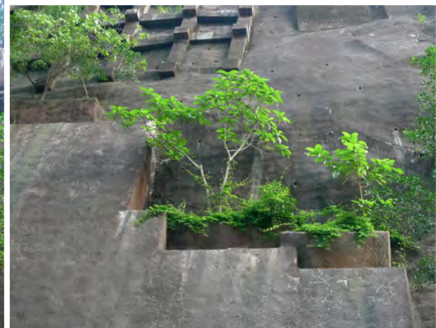
Coloured buttress and hard slope surface with planting at various levels
