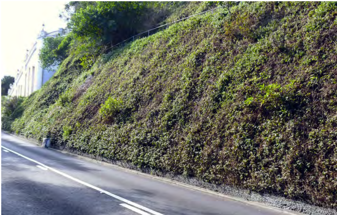
Wedelia trilobata growing in mulching panels on a hard surface
