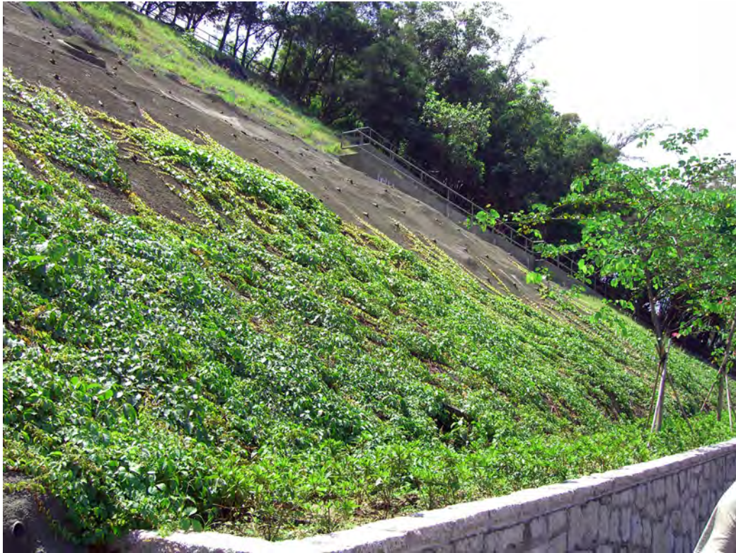
Planting of climbers in a toe planter to minimise the visual impact of a hard slope surface
