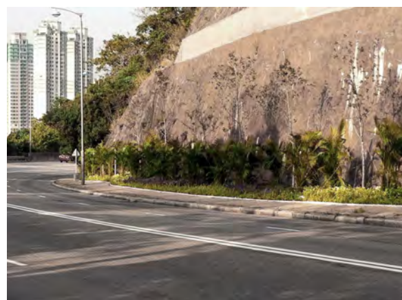
Painted slope hard surfacing further screened by planting in toe planters
