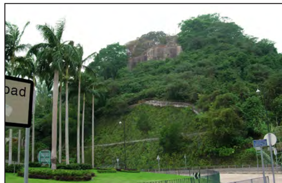
2 years after slope upgrading works (2007)
