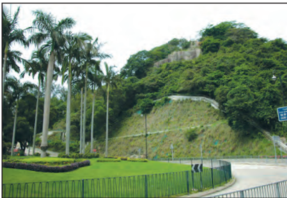
Completion of construction (2005)
