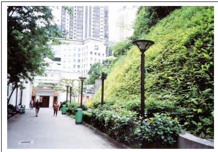
Figure 4.12 Reinforced Fill Slope with Vegetated Surface
