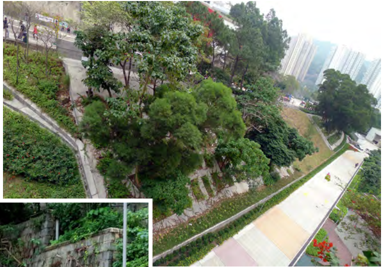
Soil nail heads encased in an irregular grillage structure for retention of existing vegetation
