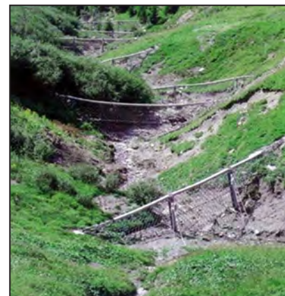
Example (from overseas) of the use of multiple flexible barriers within drainage channels
