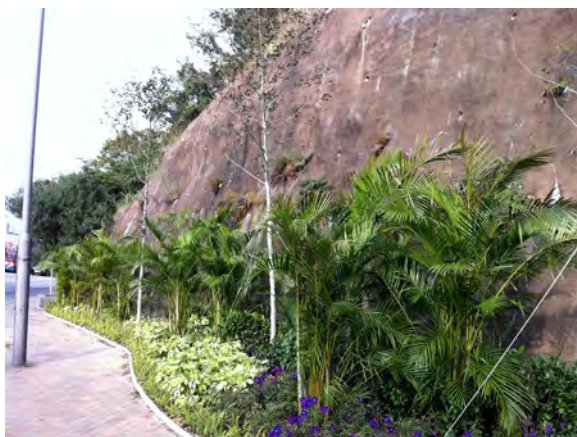
Painted slope hard surfacing further screened by planting in toe planters
