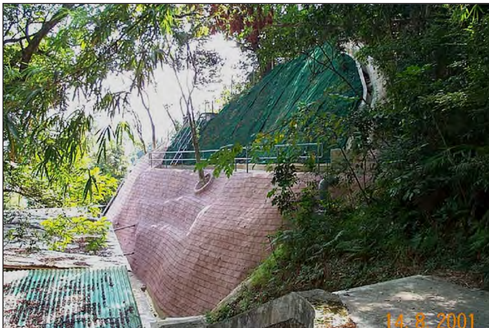
Completion of construction (2001)
