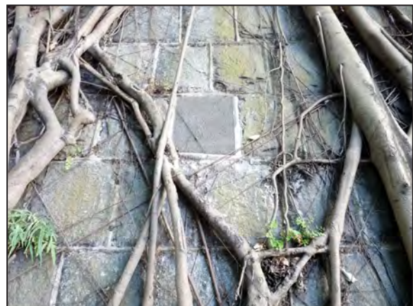
Close-up of granite texture finish to concrete soil nail head
