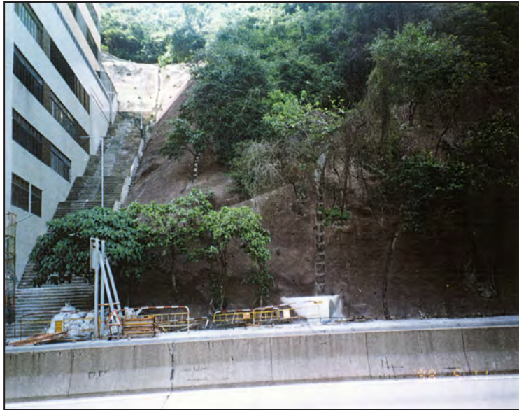
Existing cut slope before site formation works (1998)
