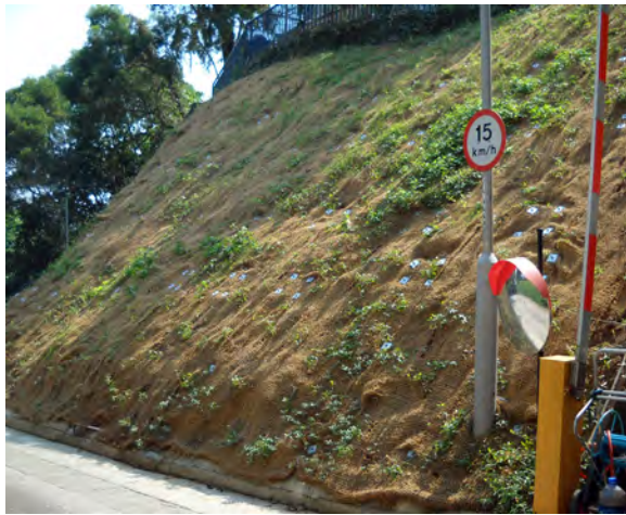
(a) Biodegradable erosion control mat
