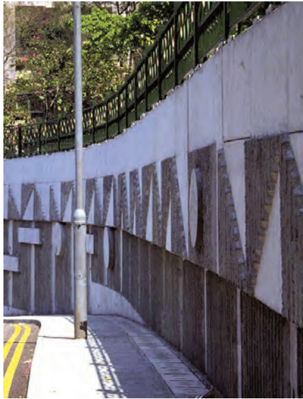
Off-formwork graphic pattern finish to RC retaining walls
