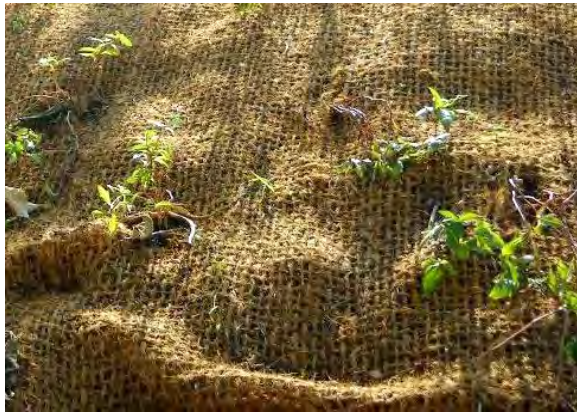
(c) Close-up of biodegradable erosion control mat
