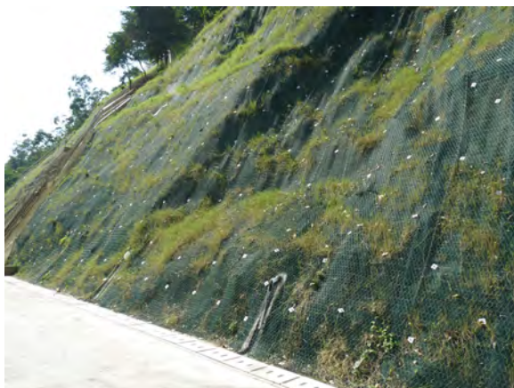
(e) Wire mesh over non-biodegradable erosion control mat
