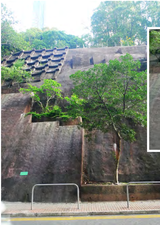
Coloured buttress and hard slope surface with planting at various levels
