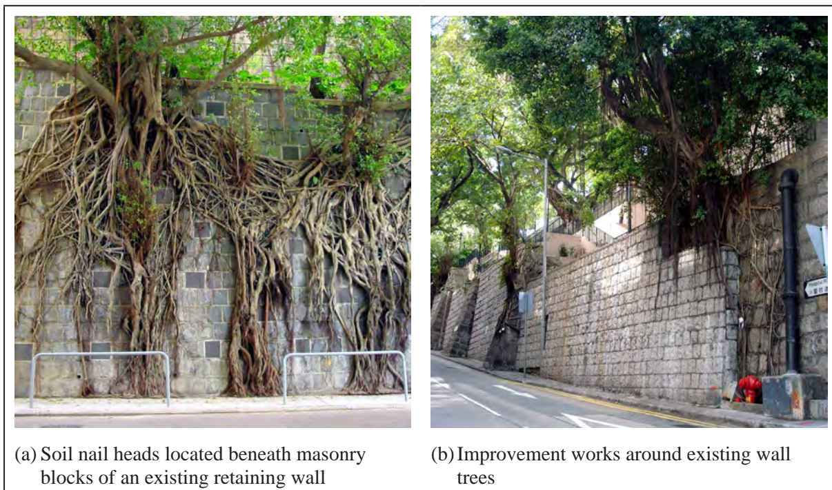
Figure 4.14 Masonry Retaining Walls with Existing Trees
