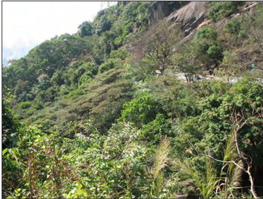
Fill slope before upgrading works (2007)
