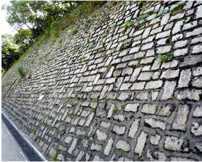
(a) Satisfactory appearance of soil nails heads beneath stone pitching
