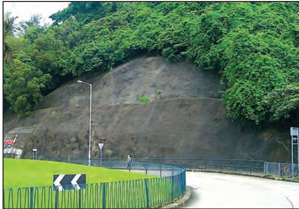
Slope before upgrading works (2001)
