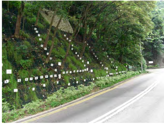
1 year after slope works with hydroseeding and pit planting of native species seedlings
