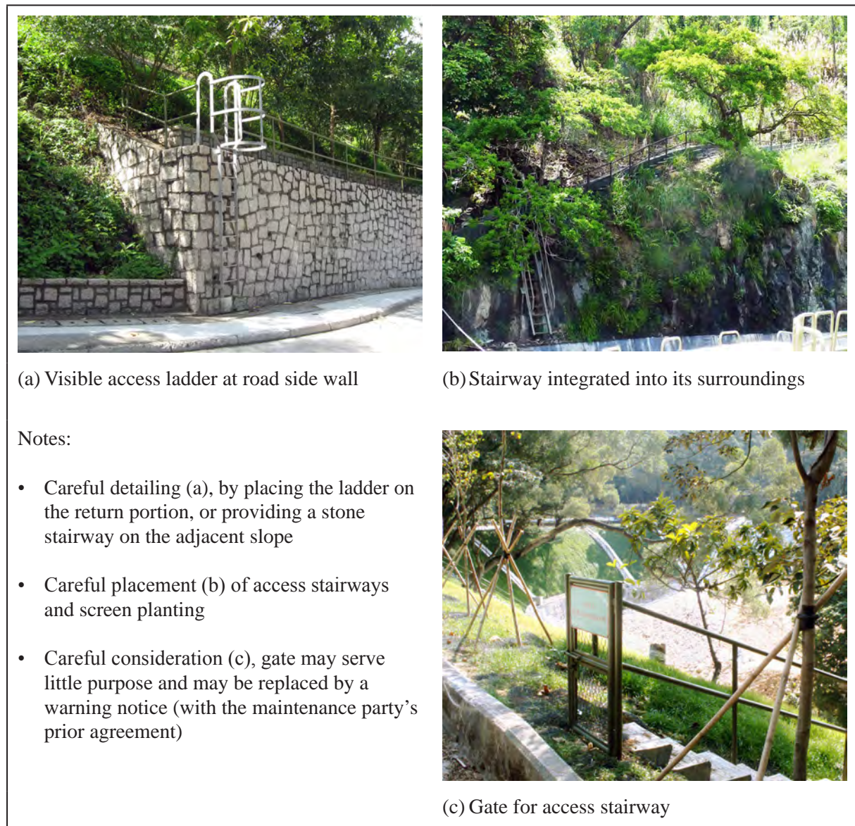
Figure 2.8 Mitigating the Visual Appearance of Maintenance Access
