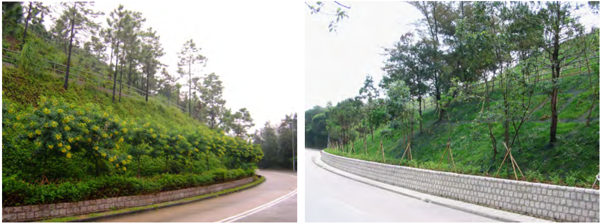
General illustrations of the use of toe planters to support planting
