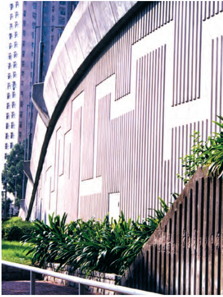
Off-formwork graphic pattern finish to RC retaining walls
