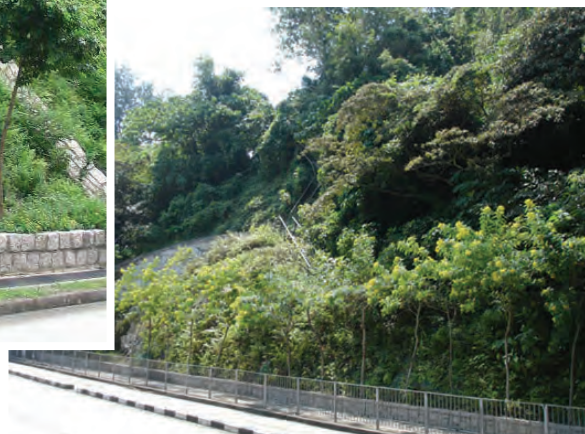
Illustration of landscaping to man-made slopes along South Lantau Road to improve visual appearance, as well as enhance ecological value by planting native species
