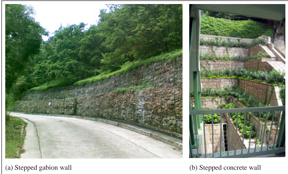
Figure 2.5 Reducing the Scale of Retaining Walls
