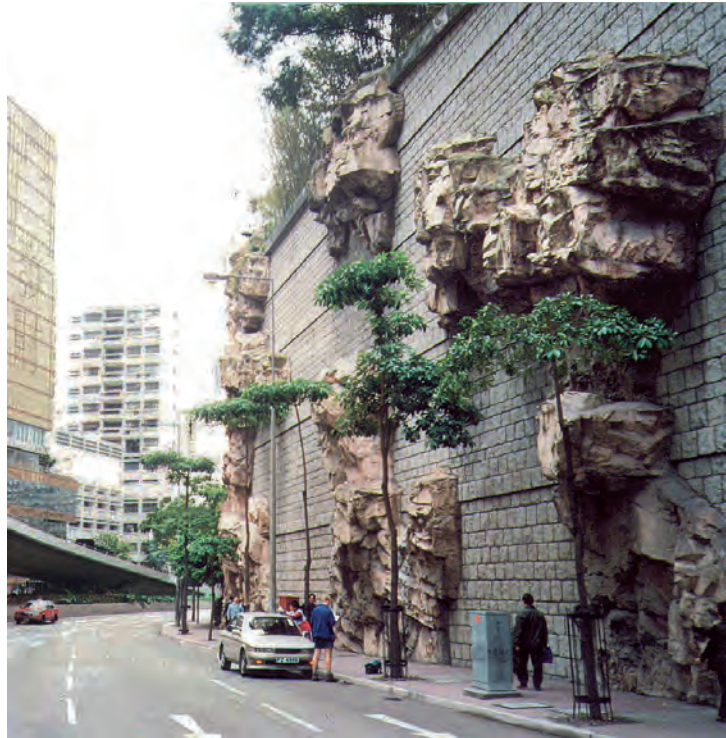
Artificial rock blocks incorporated into masonry surface finish
