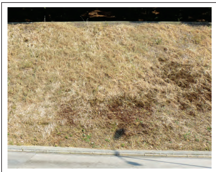
Figure 2.23 Common Appearance of a Sprayed Mulching System during Dry Season
