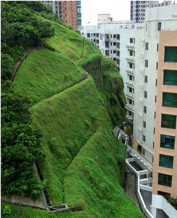
Planting on hard surfacing using proprietary mulching system on a steep cut slope
