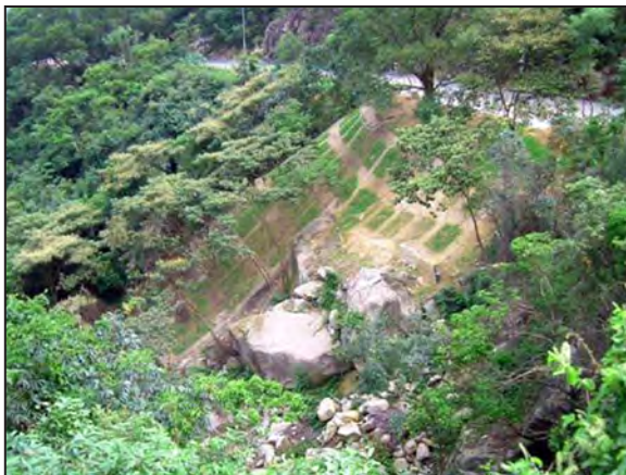
Slope upgrading works substantially completed (2009)
