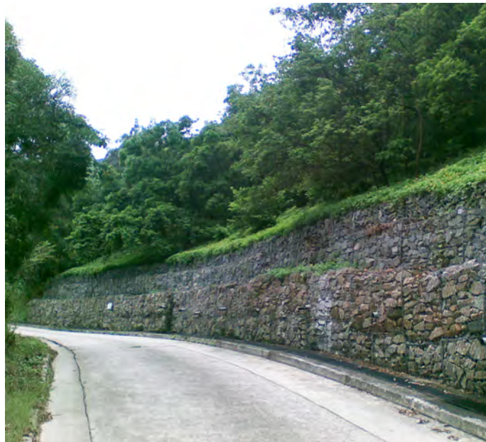
Exposed stonework appearance by the use of gabion walls
