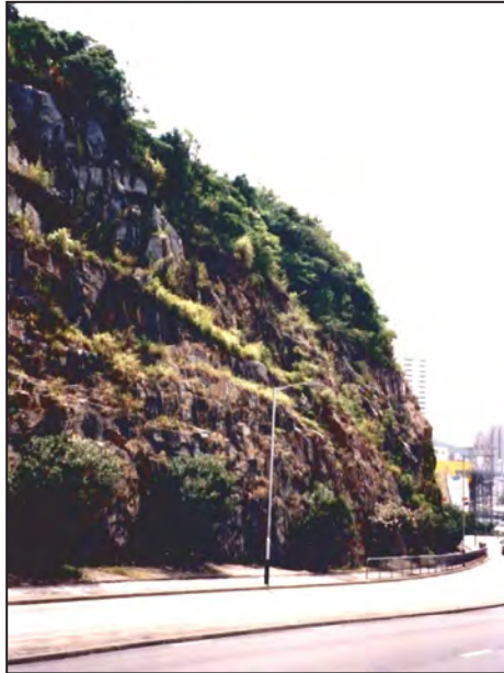
Rock cut slope before upgrading works (2000)
