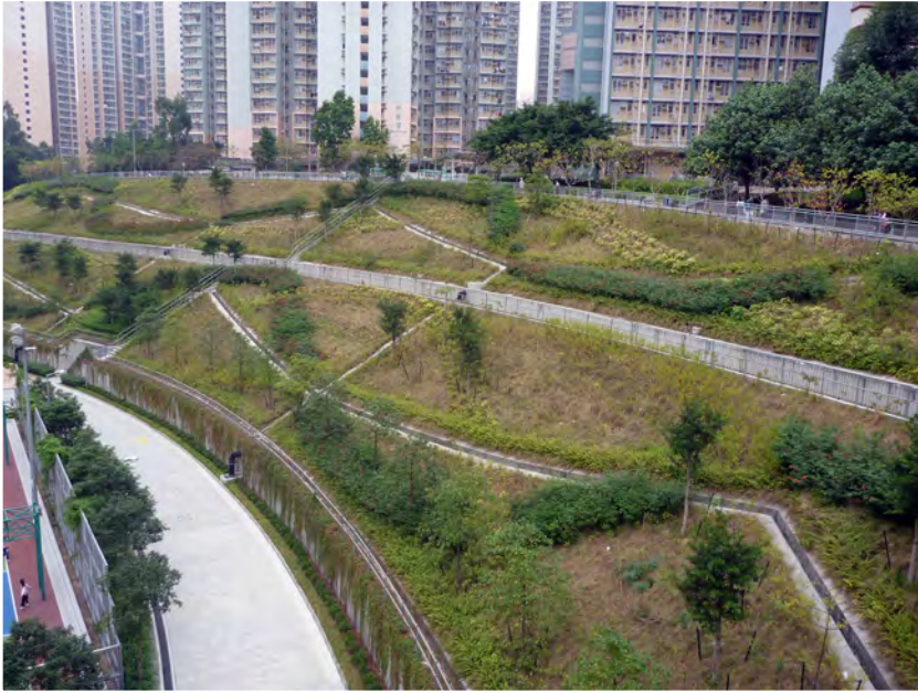
A vegetated cut slope with retaining wall at the toe (vegetation in a crest planter trailing down the wall)
