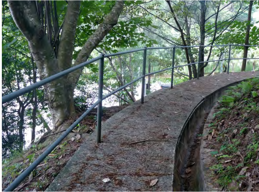
Handrails of reduced sizes and coloured to suit the site conditions
