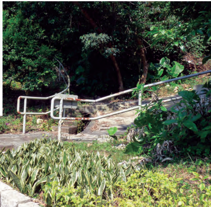
Access to maintenance stairways serving two slopes discretely placed through planter
