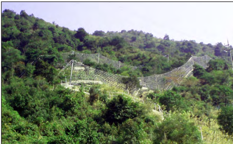
Natural terrain mitigation works completed (vegetation is beginning to screen the flexible barriers and maintenance access)
