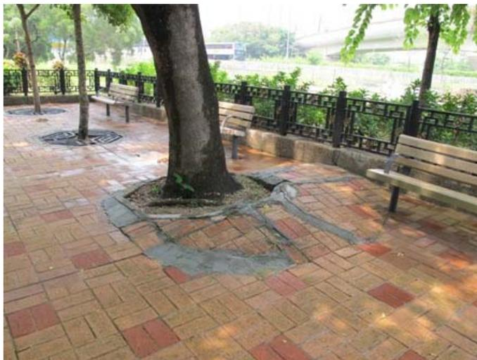
Fig. 2 Pavement lifting caused by root growth
