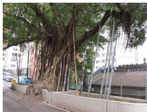
Photo 8 - Installation of guiding tubes to facilitate development of lignified aerial roots to the ground for additional supports
