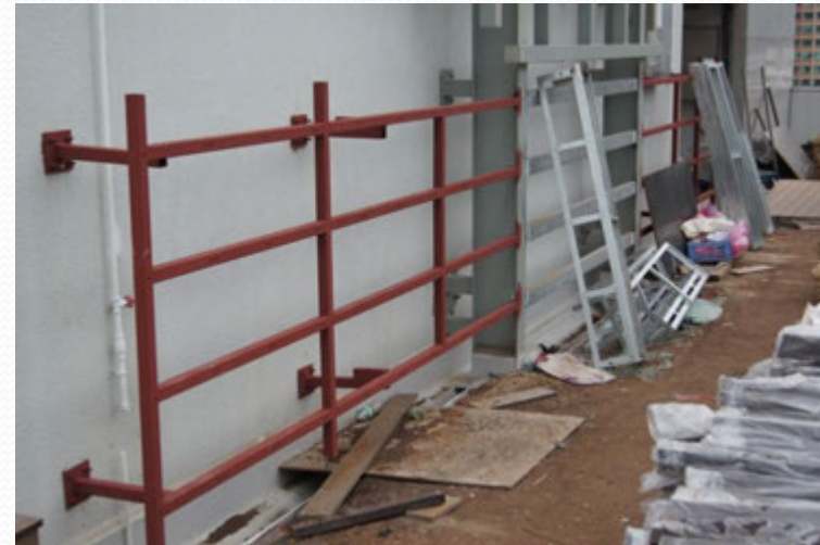
Vertical Green Wall- Sub frame
