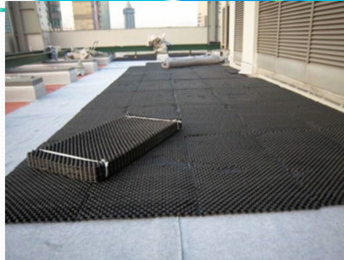
Green Roof System Installation
