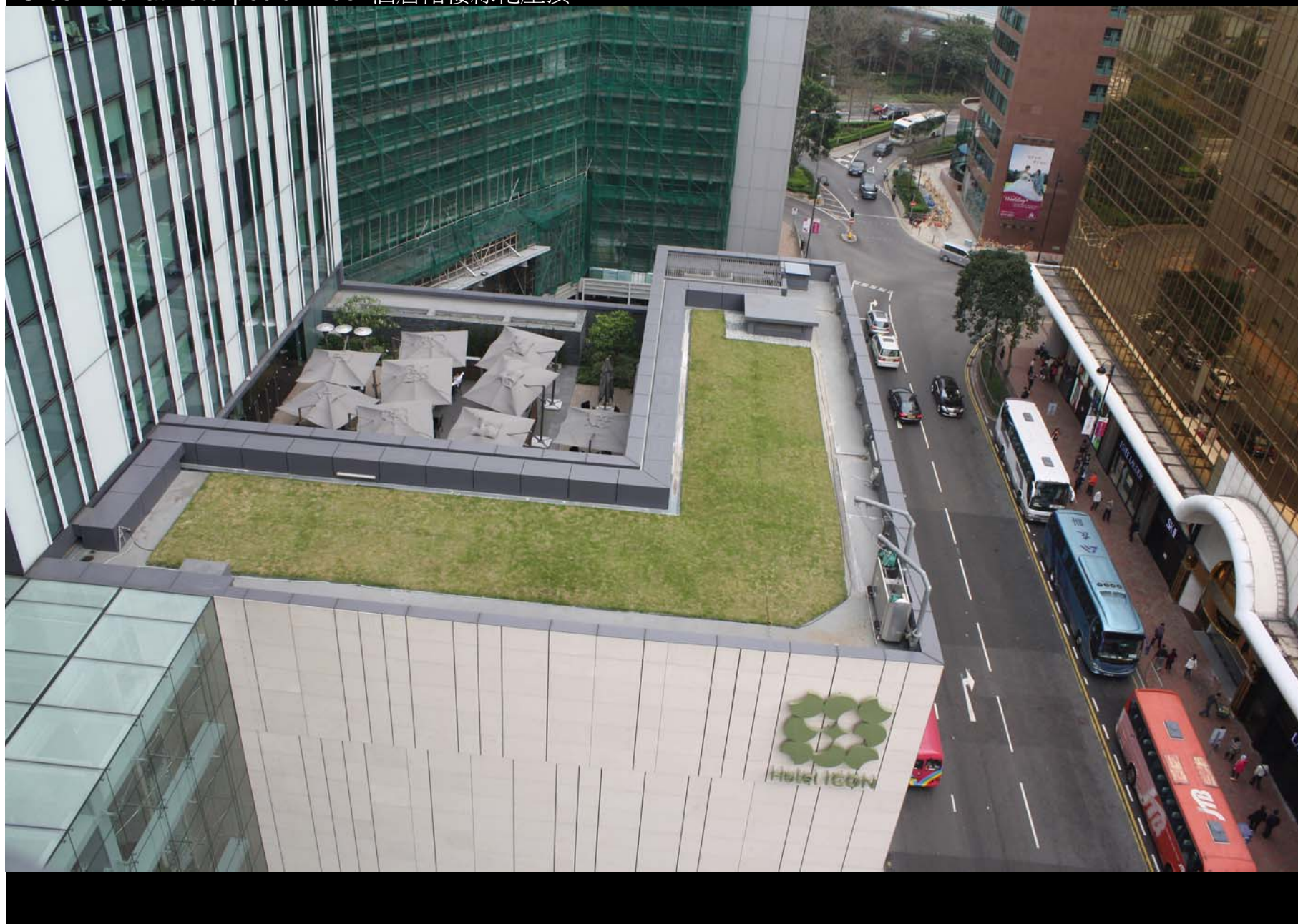
Green roof at hotel podium roof 酒店裙樓綠化屋頂
