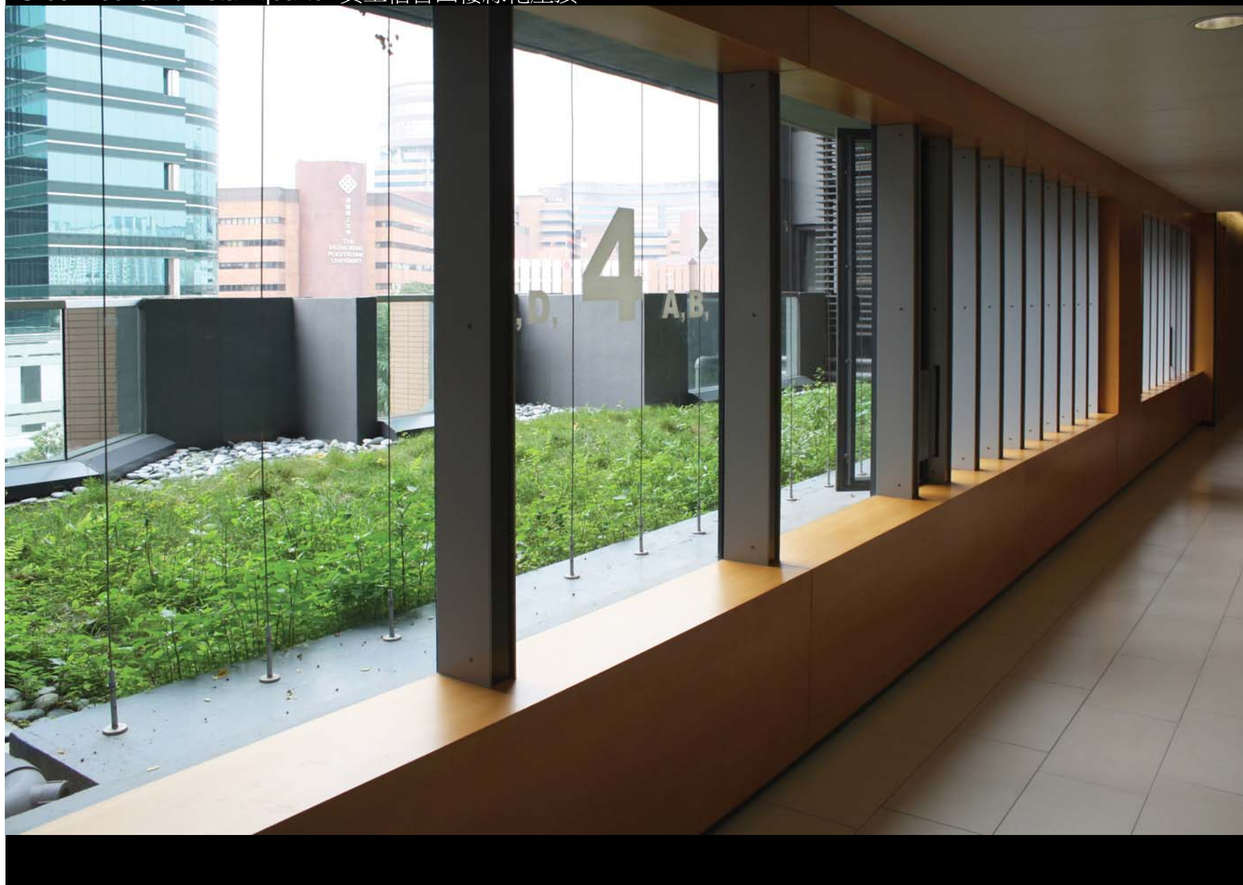
Green roof at 4/F staff quarter 員工宿舍四樓綠化屋頂
