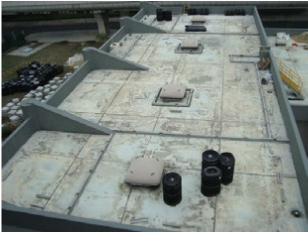
1. Clean up rooftop surface
