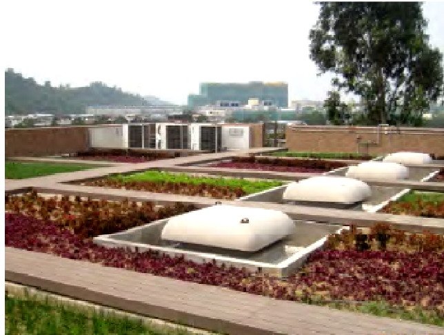
Kau Hui Pumping Station
