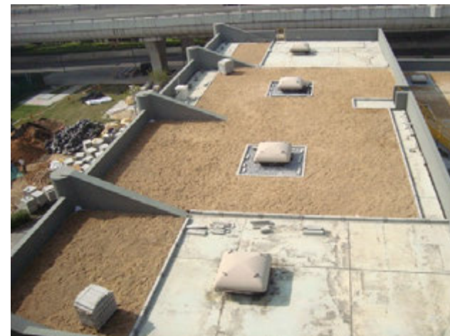
5. Placing planting soil
