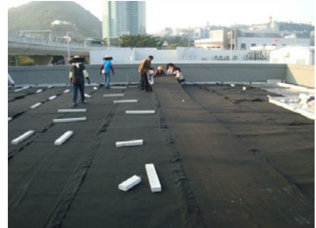
3. Install drainage composite layer
