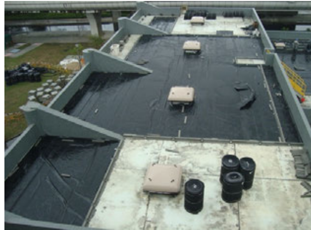
2. Install root barrier
