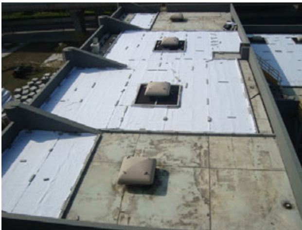
4. Install water retention mat
