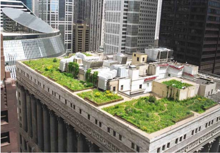
The Chicago City Hall (Its green roof helps cool the building and minimize water run-off.)
