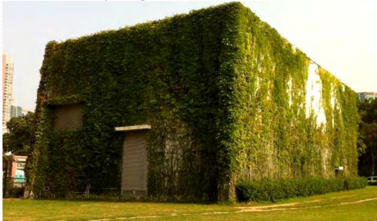
Tai Hang Tung Floodwater Pumping Station
