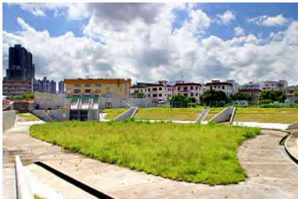
Village flood protection scheme in Ma Tin Tsuen, Yuen Long
