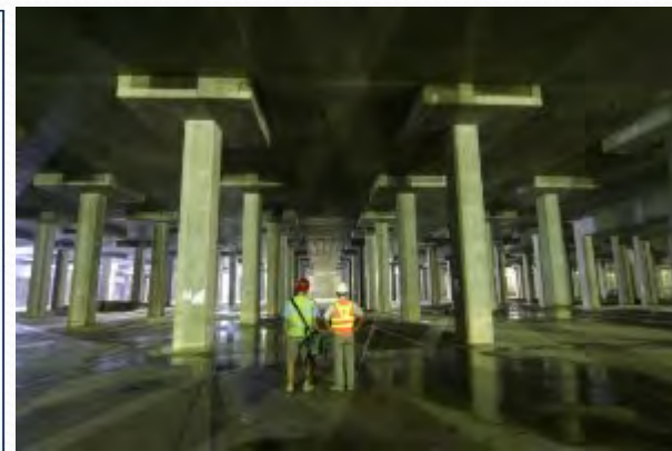
Tai Hang Tung Stormwater Storage Tank
