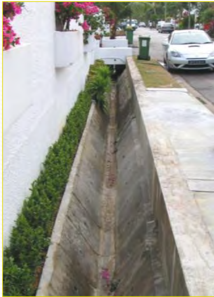
Open roadside drain
