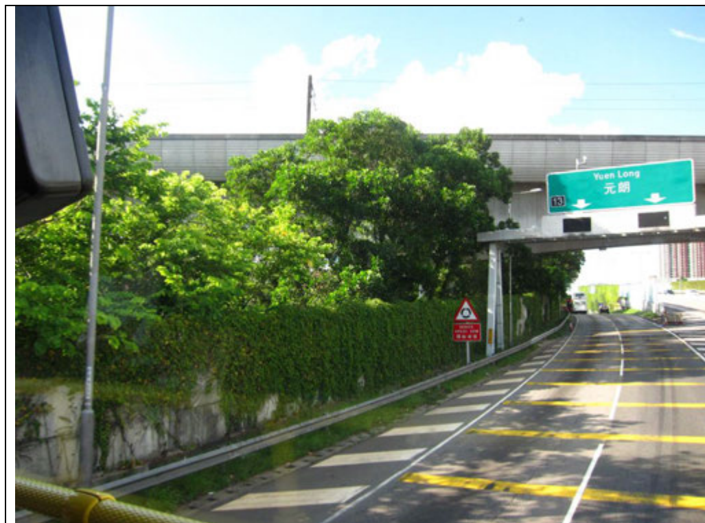
Figure 2 - Noise barrier blends into the immediate environs
