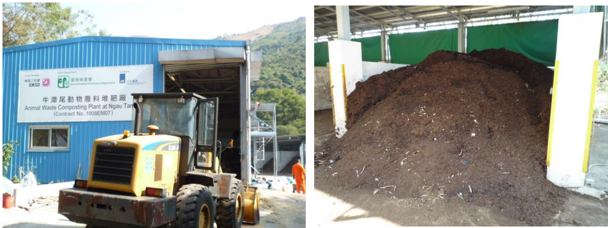
The composting plant in Ngau Tam Mei (AWCP) co-composts animal waste with yard waste and occasionally with food waste
