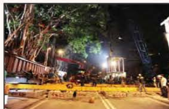
Temporary Track System
