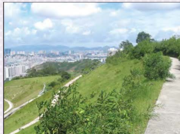
Quarry after rehabilitation (Anderson Road Quarry)
