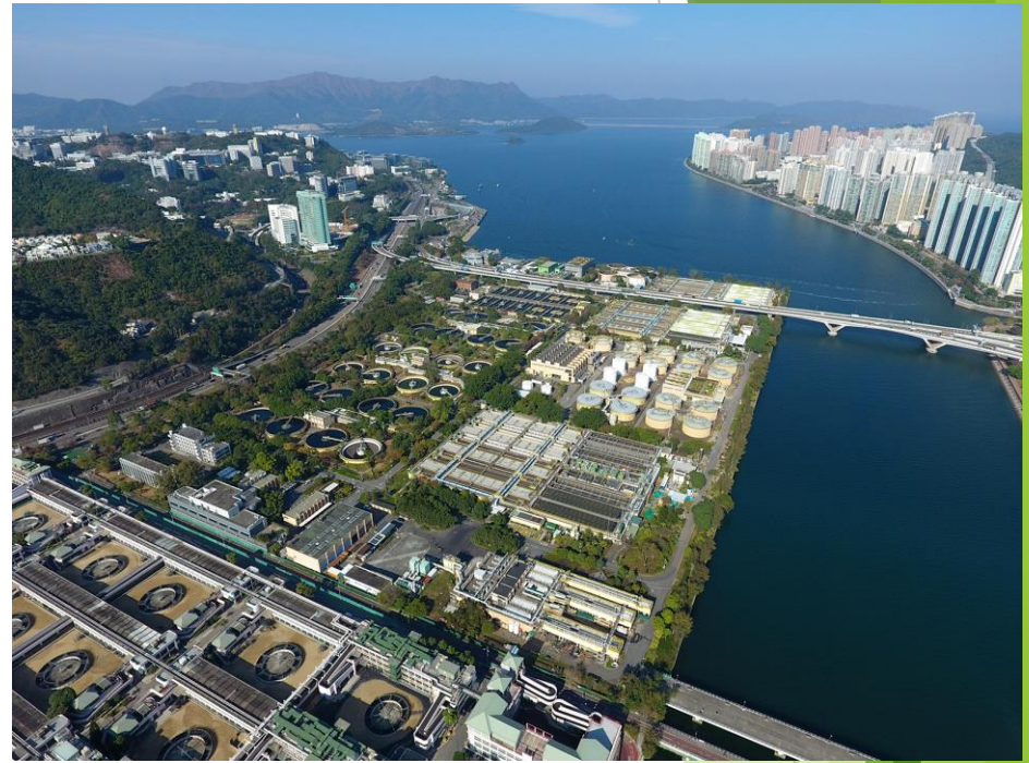
Shatin Sewage Treatment Works (internet image)
