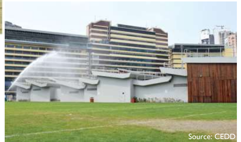
RAINWATER HARVESTING SYSTEMS
